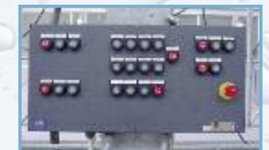
Remote control at the wash bay, fully explosion proof.
