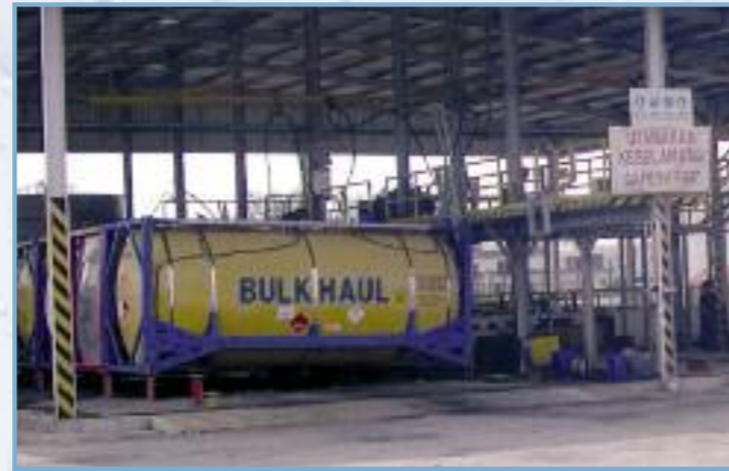
Washing channel in Malaysia.
