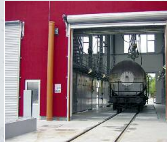
Tank internal cleaning plant for the Croatia Railway.
